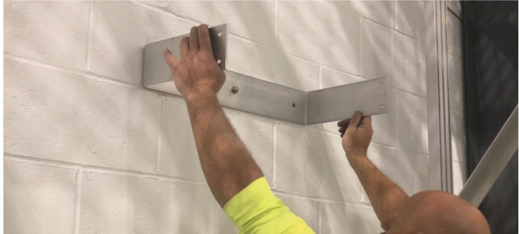
Hold the bracket in position and mark the center hole. Remove the bracket and drill the center hole using a 1/2in masonry drill bit. Position the bracket and insert a 1/2in S/S Sleeve Anchor into the center hole. Hand tighten. With the bracket held in place and level, drill the remaining (2) holes through the pre-drilled holes with the 1/2in drill bit. Initially drilling through the wall bracket will ensure accurate hole placement.
