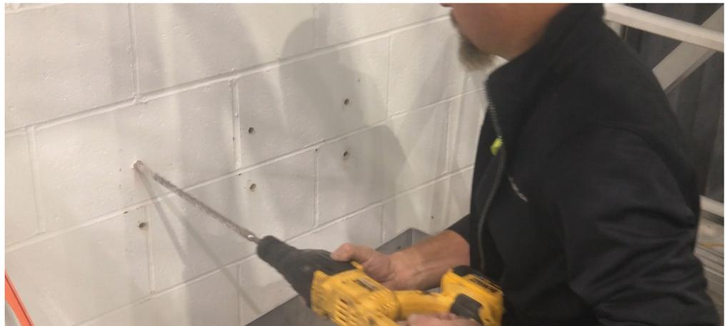
Once the 1/2in holes are drilled, remove the wall bracket and using a 5/8in drill bit, re-drill the (4) outer holes. Once drilled, blow out the debris and insert the mesh sleeve and close the cap. Mount the bracket using the (2) 1/2in S/S Sleeve Anchors in the center holes.
