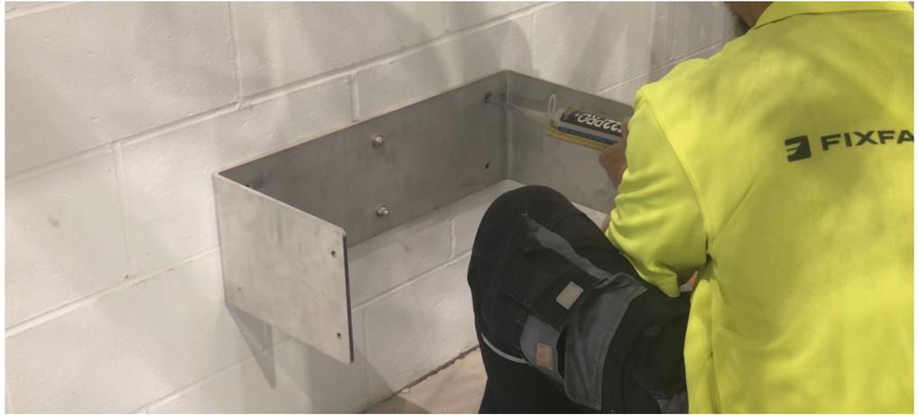
Fill the (4) outer holes with EP1001 VF22 Epoxy. Insert the 3/8in S/S Stud into the (4) outer holes giving it a 1/2 turn as you insert. Then let the epoxy cure as per the instructions below. Remember weather can affect the cure time.
