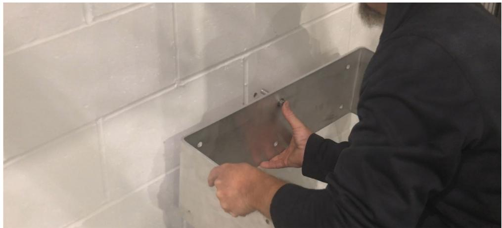
Hold the bracket in position and mark the 2 center holes. Remove the bracket and drill the top hole initially using a 1/2in masonry drill bit. Mount the bracket and insert a 1/2in S/S Sleeve Anchor into the top hole. Just hand tighten as the bracket will need to be removed again. With the bracket held in place and level, drill the remaining (5) holes through the pre-drilled holes with the 1/2in drill bit. Initially drilling through the wall bracket will ensure accurate hole placement.
